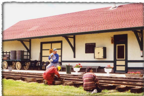
Track being laid in front of station.
