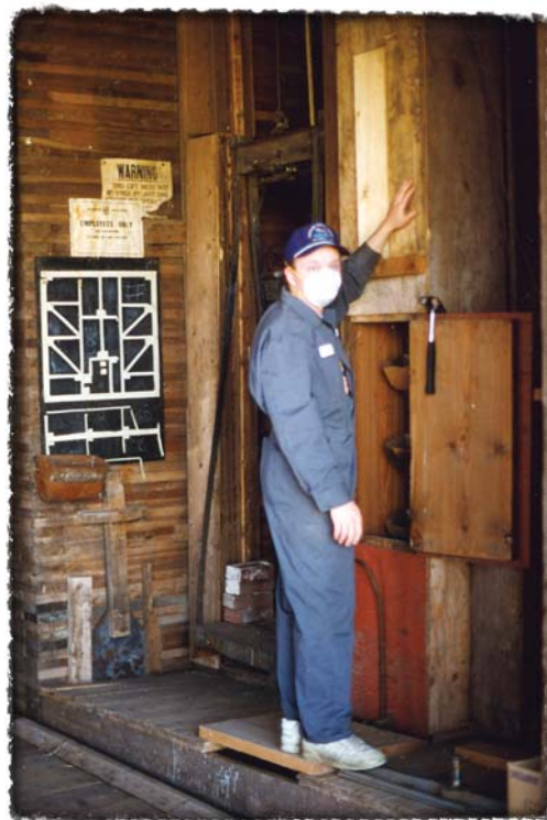
Restoration work started in the Meeting Creek AB Pacific elevator, 1999.
