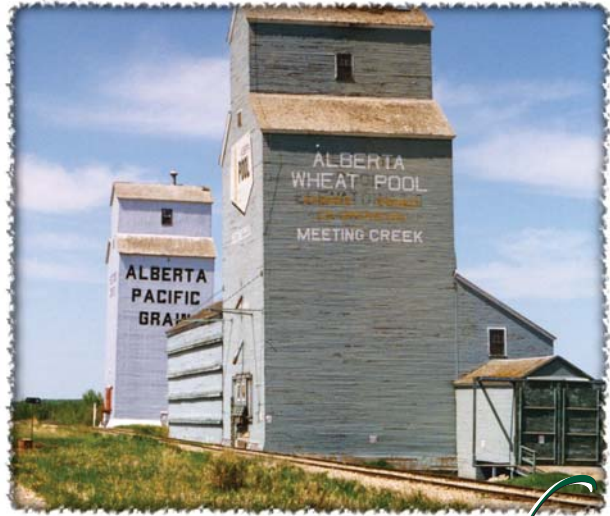
Meeting Creek elevators before restoration work started, 1987.
