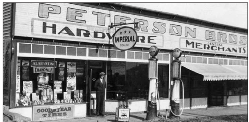
Meeting Creek in the 1930s—Peterson Brothers Hardware store, located on Main Street, had a thriving business serving local needs. Photo courtesy of Jerry and Lorene Bergstrom of Meeting Creek.
