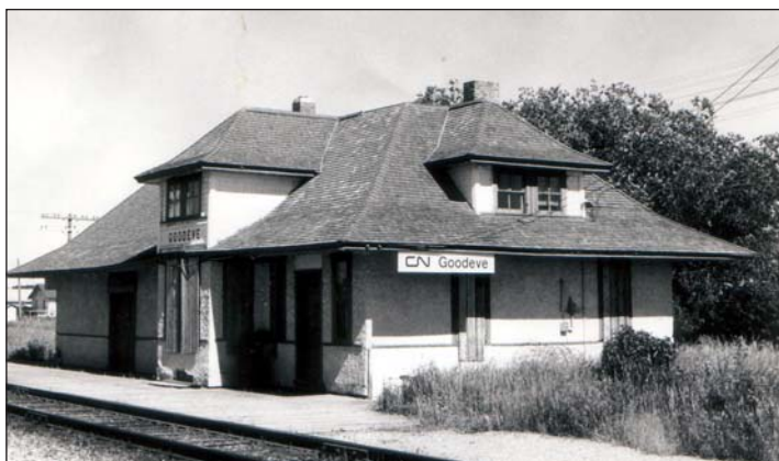
Goodeve, SK, GTP depot, looking NW, August 1971. Depot was built in 1909.
