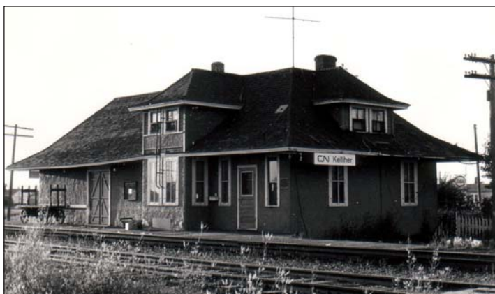
Kelliher, SK, GTP depot, looking NW, August 1971. Depot was built in 1909, stucco added in 1922 and plumbing in 1966. Kelliher is the hometown of our Chronicle newsletter designer and current CNoS President, Lorrie Tiegs.
